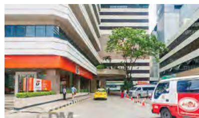
BB Buildingの外観
